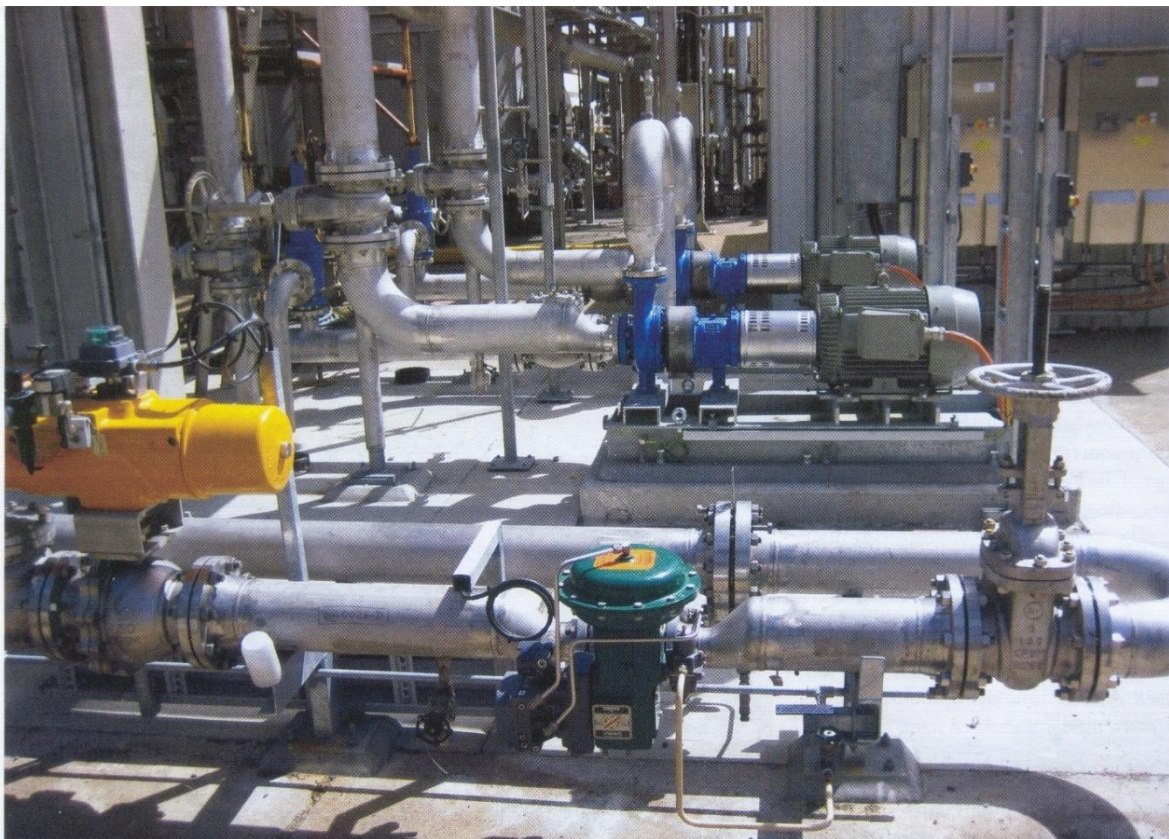
Figure 1—A Centrifugal Pump Set Installation
